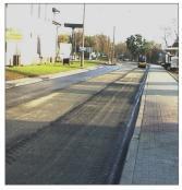
S&P Carbophalt® G installed onto bitumen tack coat.
