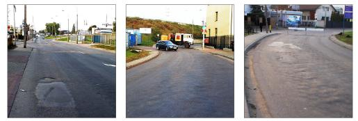
Visible damage on the wearing course, where even the pattern from the underlying hexagonal paving blocks can be seen.
