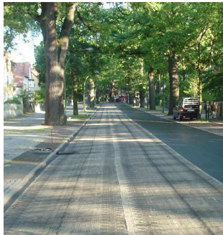
▲ Installed asphalt grid
